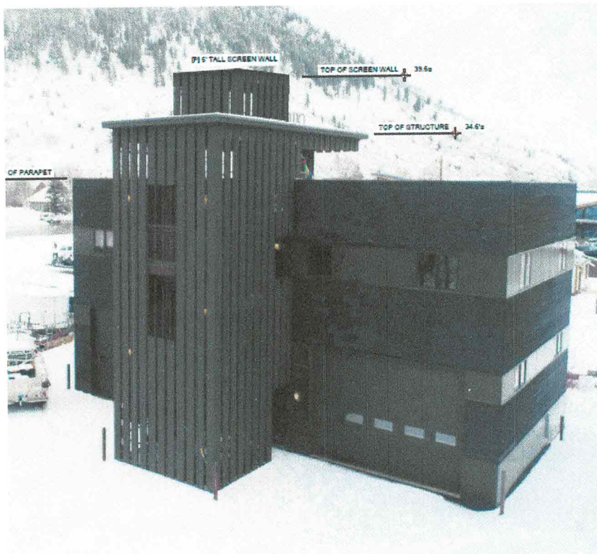
Figure 6: Proposed Stealth Screen Roof-mounted Structure for two sectors
