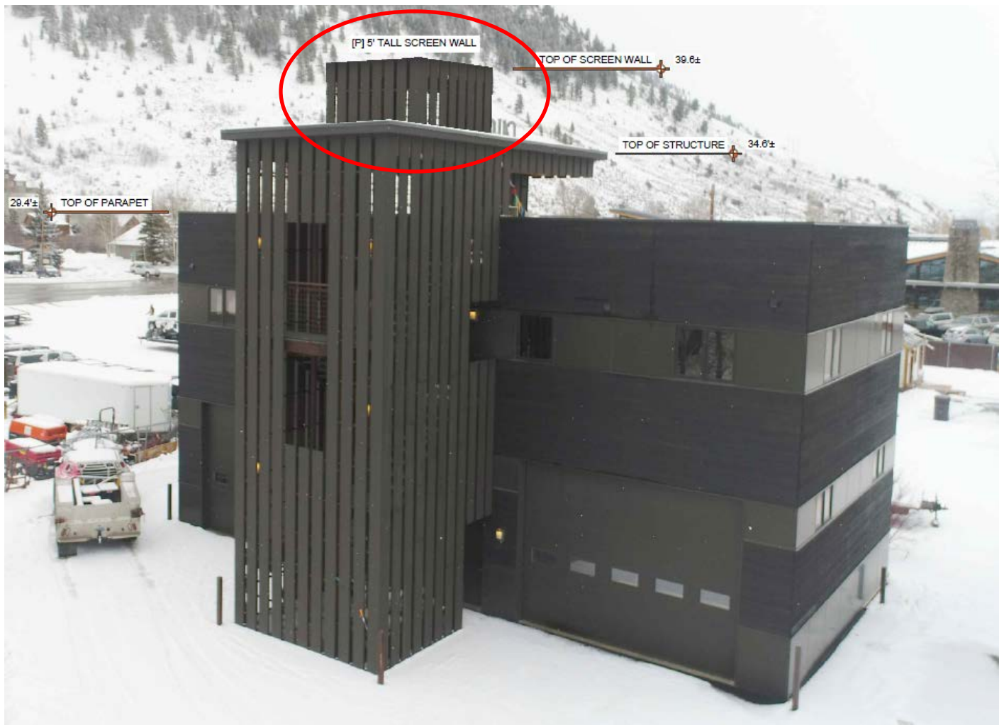
A rendering of the proposed roof-mounted 'stealth' structure as approved by the DRC.
