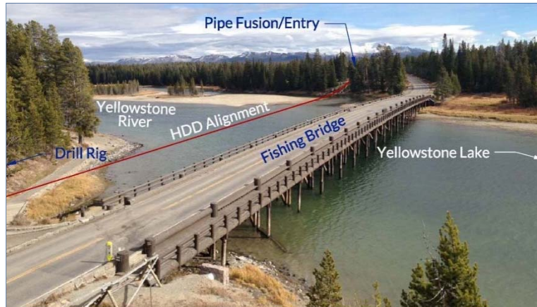
Fishing Bridge Water System HDD under the Yellowstone River, Yellowstone National Park, WY
