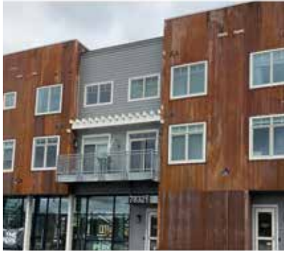
Two images selected as "Inappropriate" for Subarea 1.2
