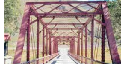
Bridge Structure - Tourism Era
