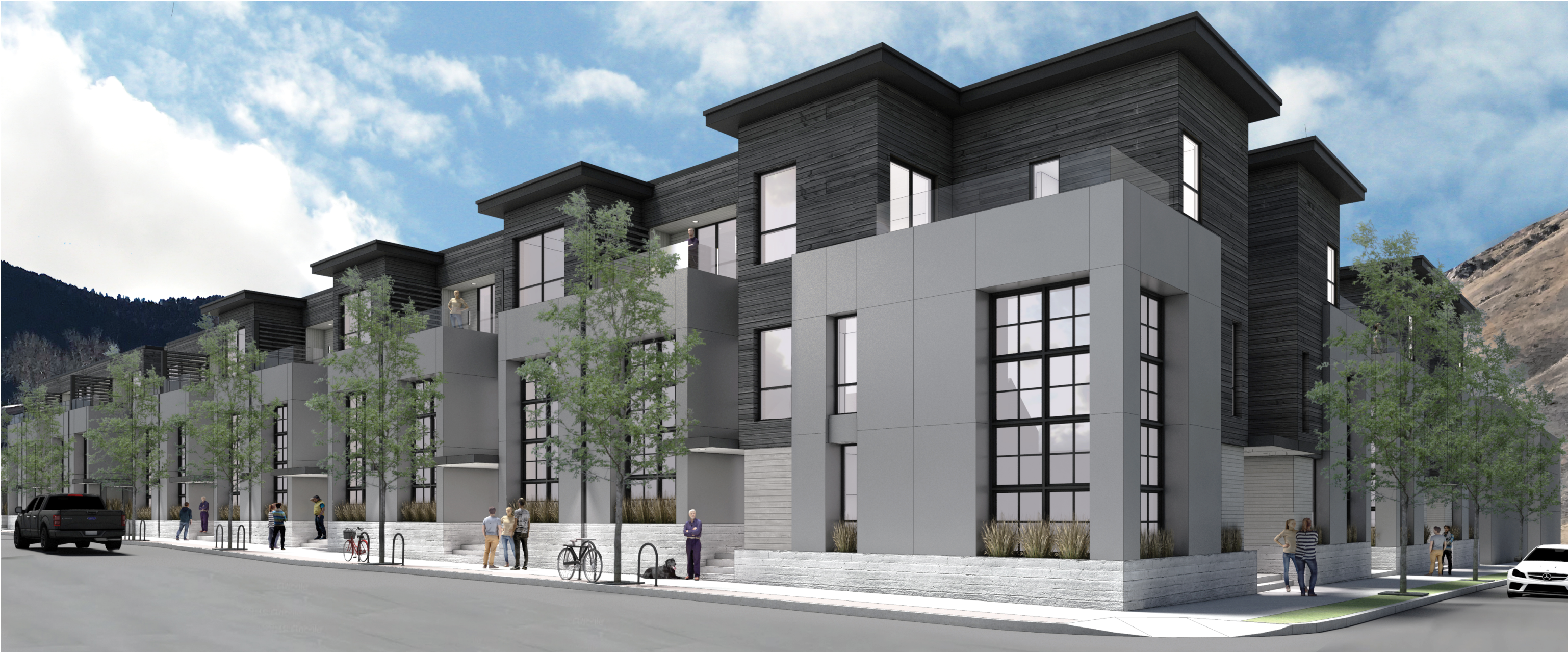
INTERSECTION OF GLENWOOD STREET & GILL AVENUE
