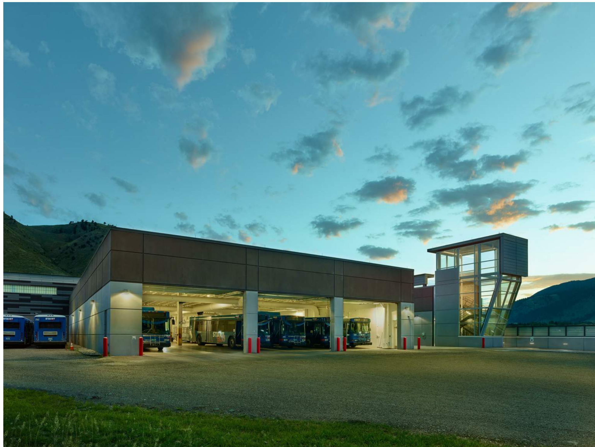
VIEW OF BUS STORAGE
