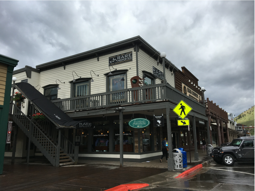
PHOTO 2 - VIEW LOOKING WEST ON BROADWAY TOWARD SUITE 1A
