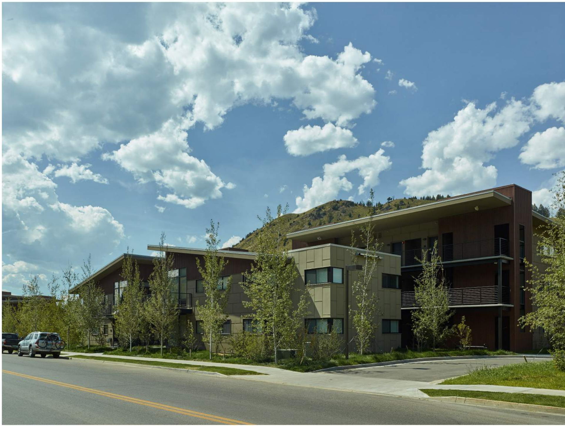
1 EXISTING FROM NORTH EAST
