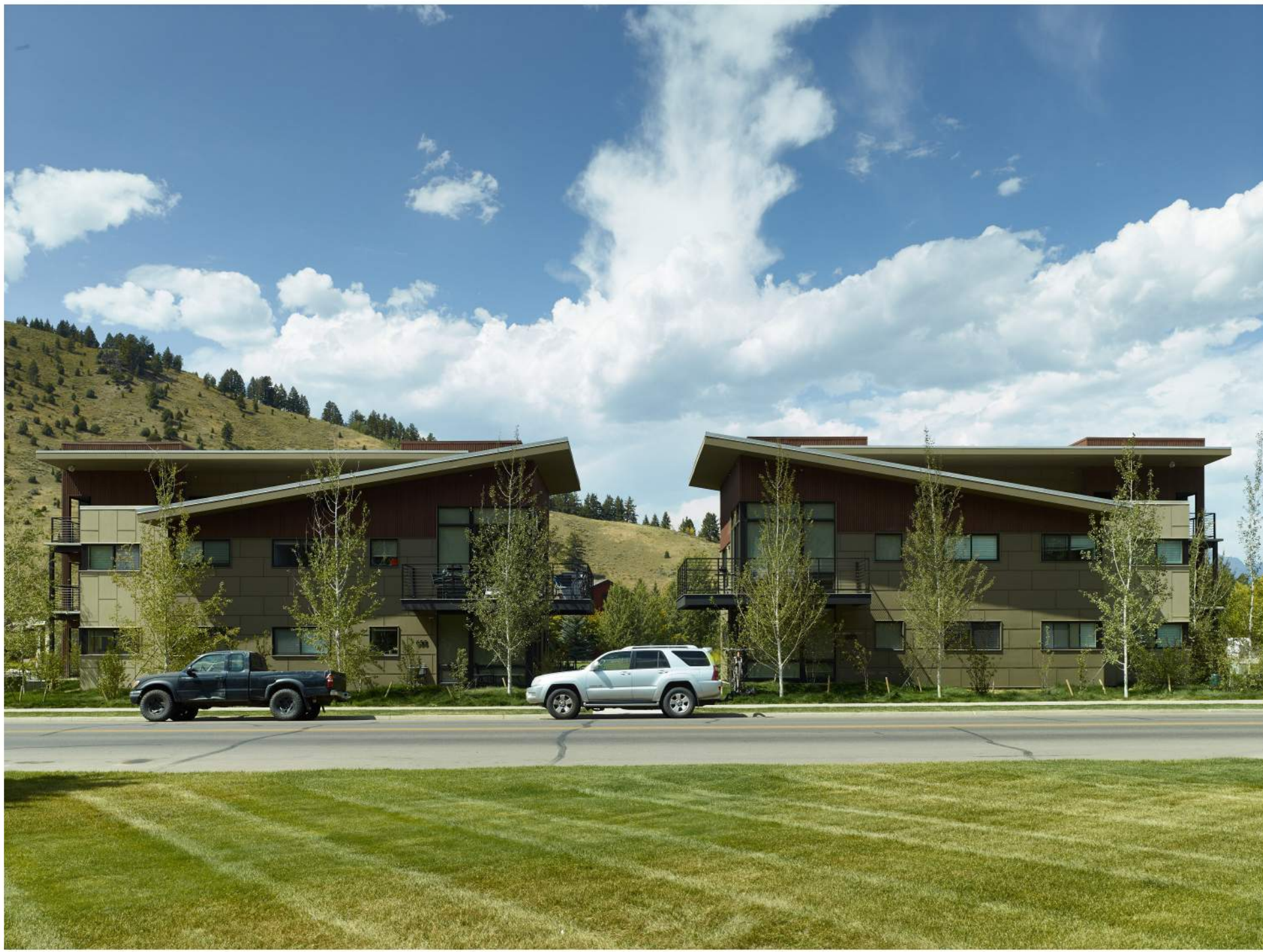
2 EXISTING FROM EAST
