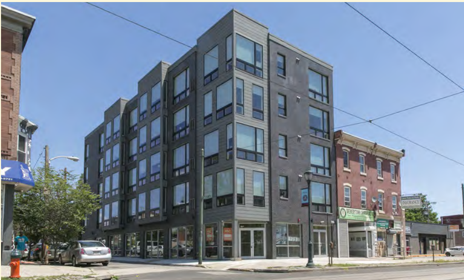
Braverman Building, Philadelphia PA
