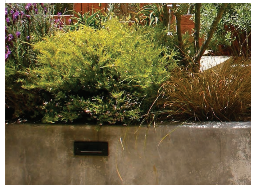
Concrete Planters at Patios
