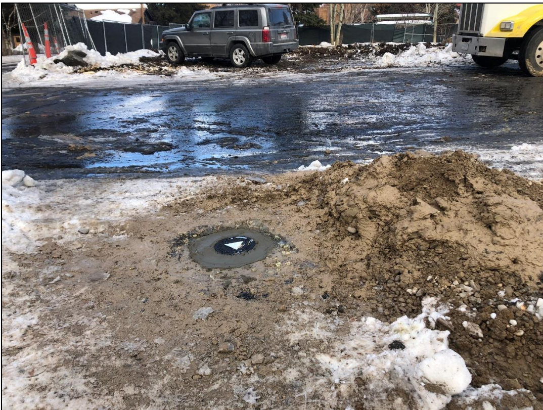
Figure 2: BH-2 Monitoring well
