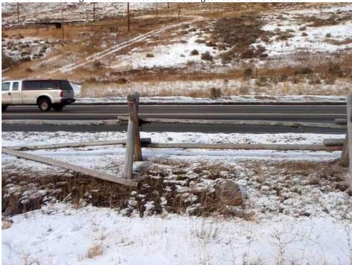
PHOTO 22 – Looking north at Broadway/HWY89 and lower face of East Gros Ventre butte.
