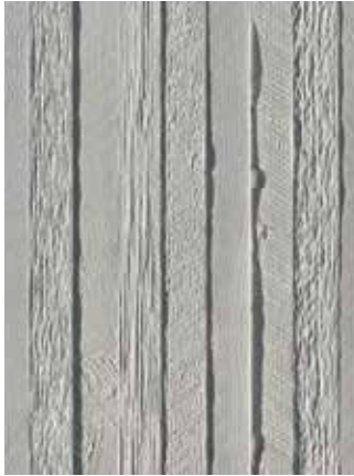
Formed concrete (wood-like)
