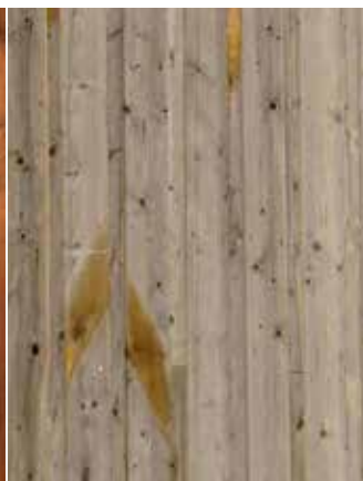
Vertical boards (weathered)
