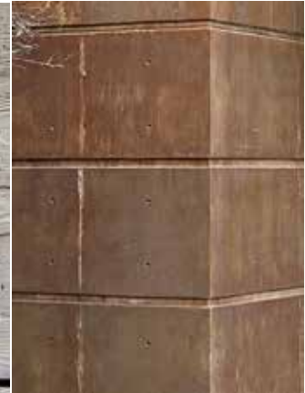
Formed concrete (colored blocks)
