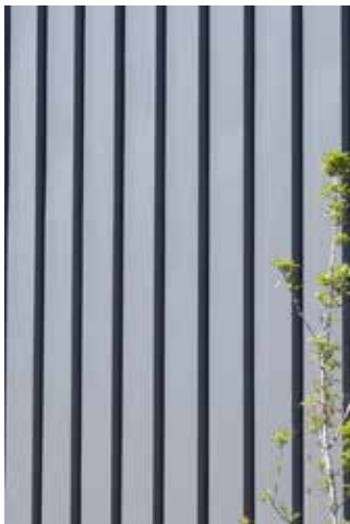
Metal panel (crimped battens)
