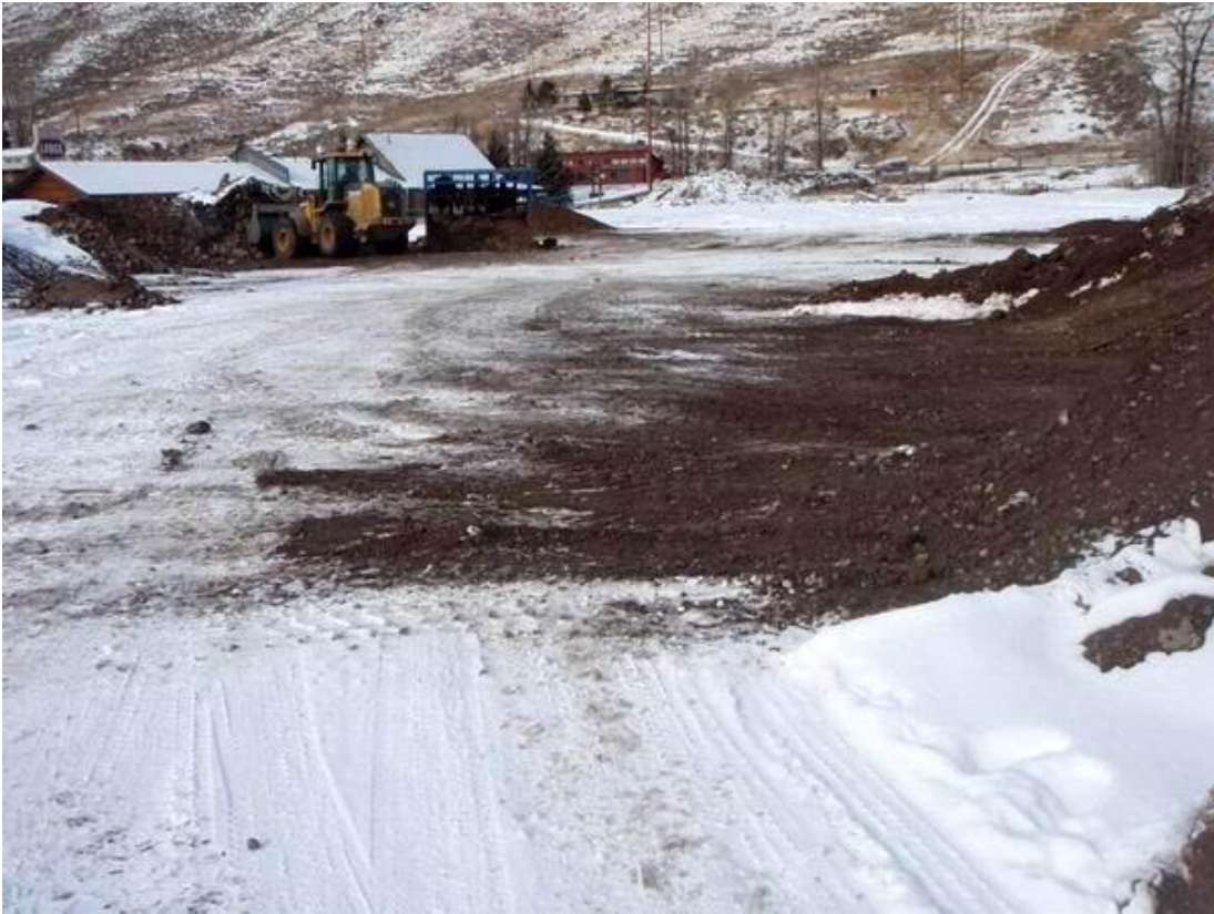
PHOTO 11 – Looking north at subject property. Disturbed ground is being used to stockpile and screen earthen material.
