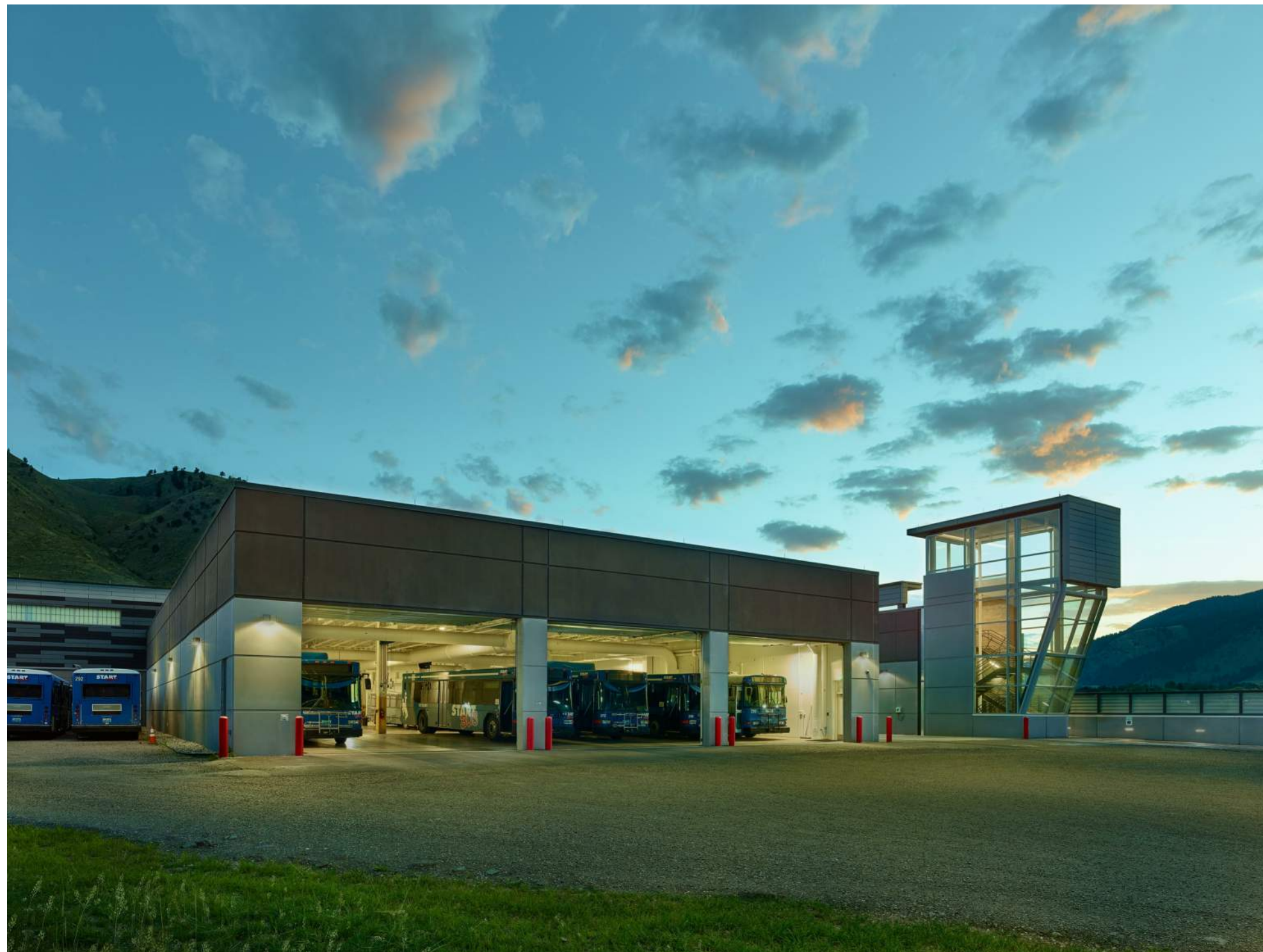
VIEW OF BUS STORAGE
