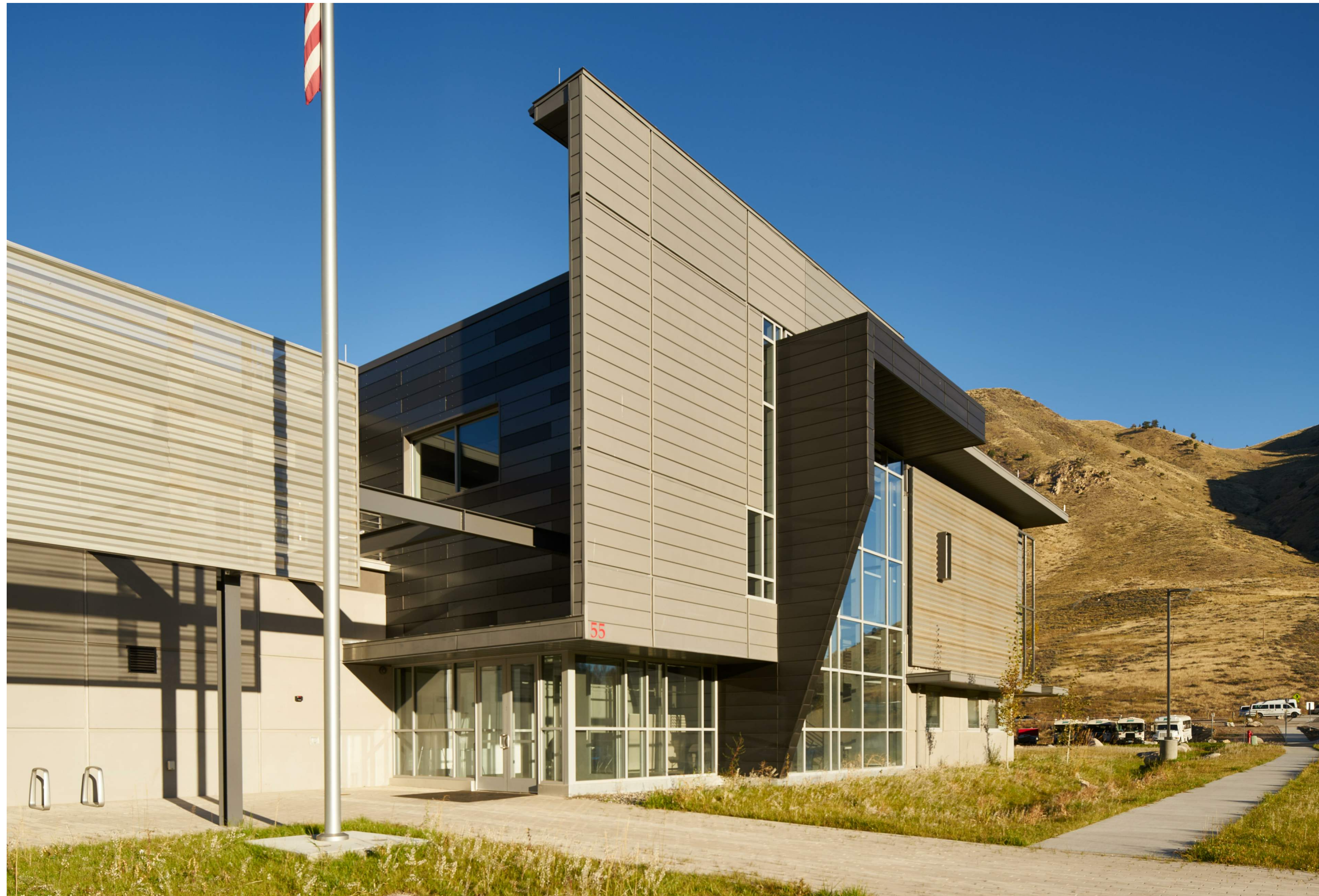
EXISTING PHASE 1 CONSTRUCTION
