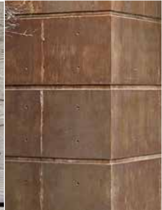
Formed concrete (colored blocks)
