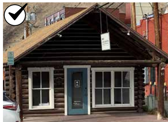
Preserve the size, position and proportion of key door openings on the primary façade.
