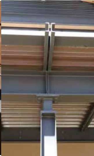
Framing connections
