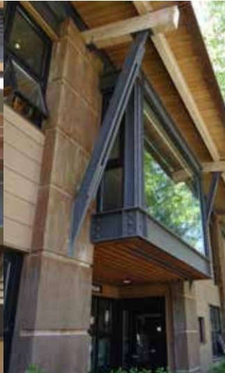
Framing connections
