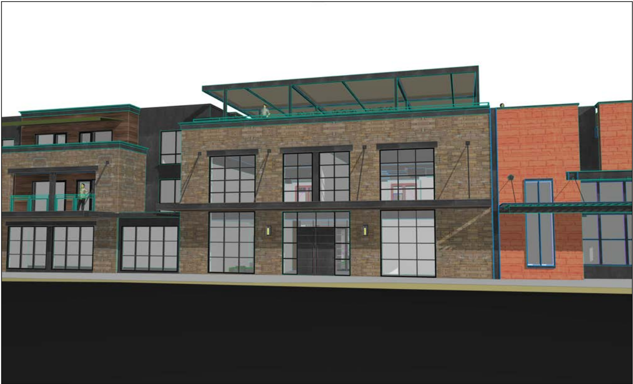
From Across Center Street
