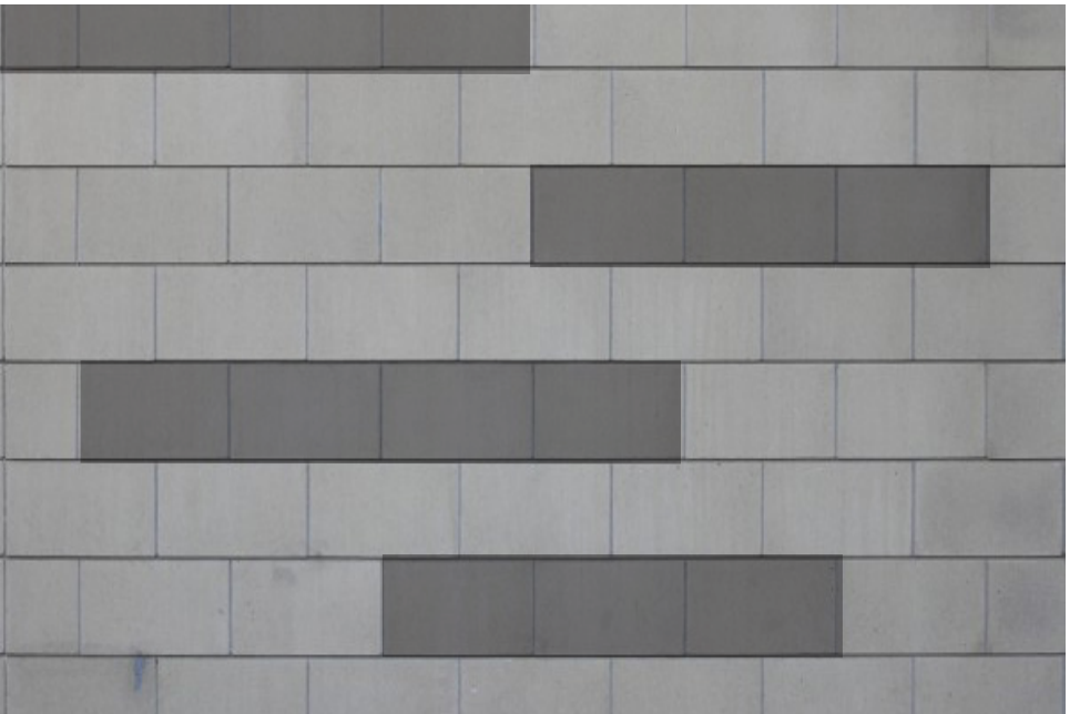
CMU - INTEGRALLY COLORED WITH HONED ACCENT BLOCK - COLOR TO BE SELECTED BY ARCHITECT
