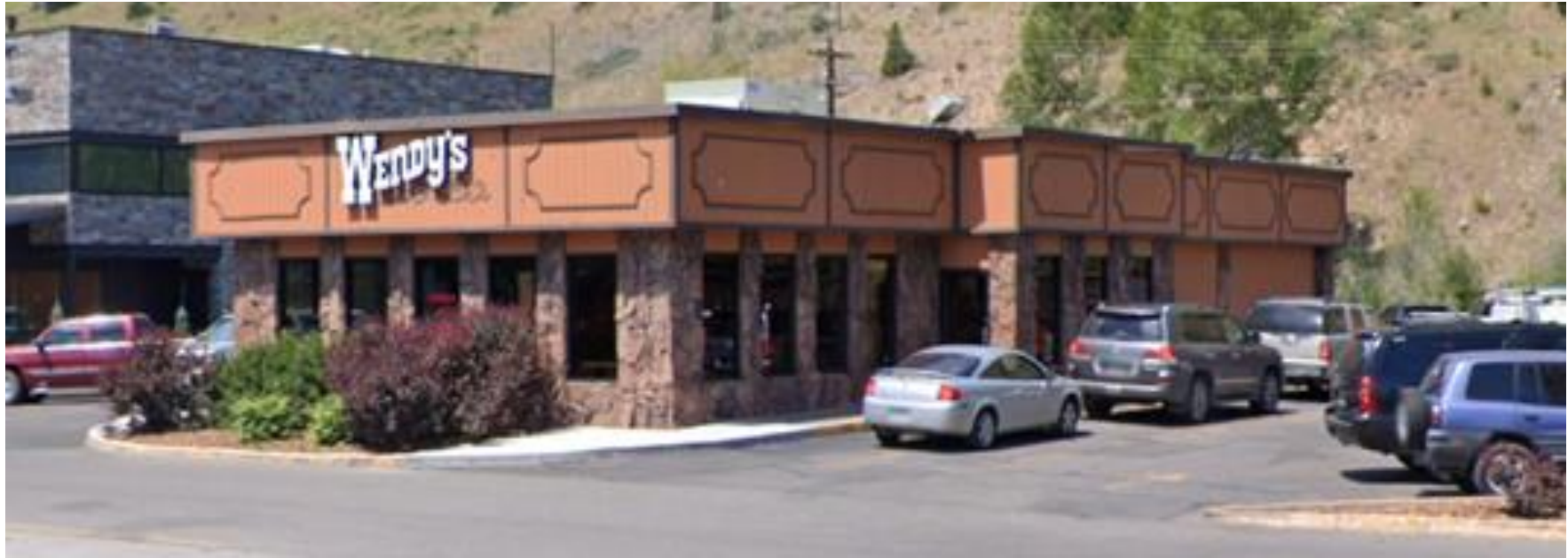
EXISTING EXTERIOR FINISHES AT WENDY'S 525 W. BROADWAY
