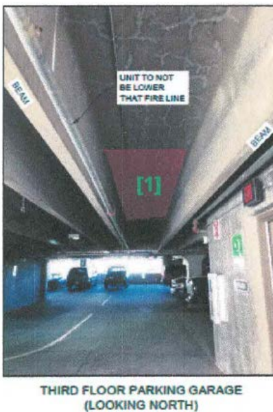
Figure 4: Proposed location for AT&T's HVAC equipment
