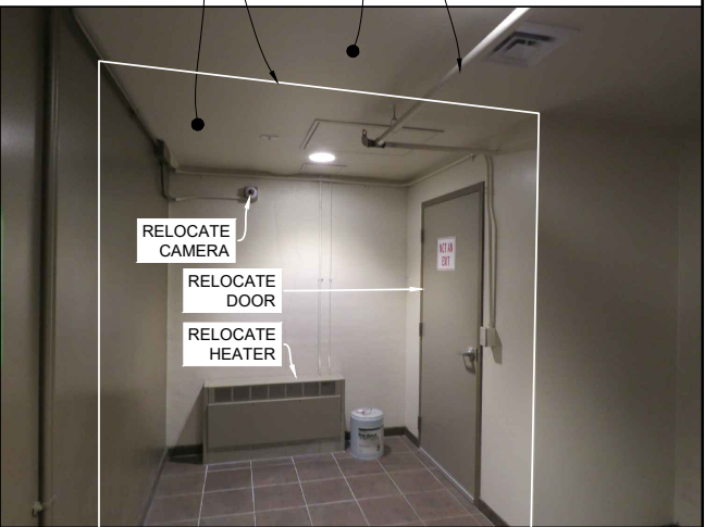
THIRD FLOOR ELEVATOR ROOM
