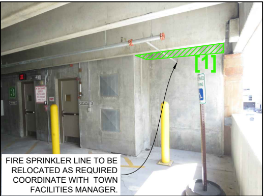
THIRD FLOOR PARKING GARAGE
