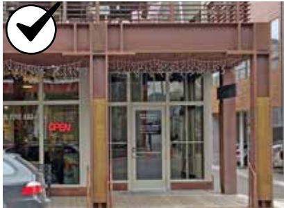
Area 1 & 2 Covered walkway
