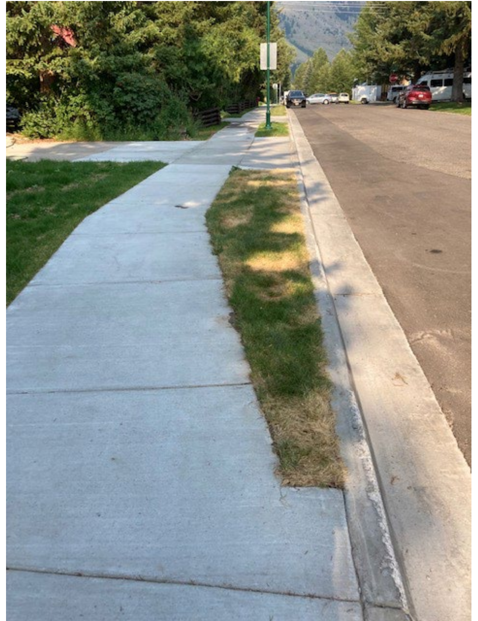
Newly sodded Kelly Ave sidewalk completed last summer
