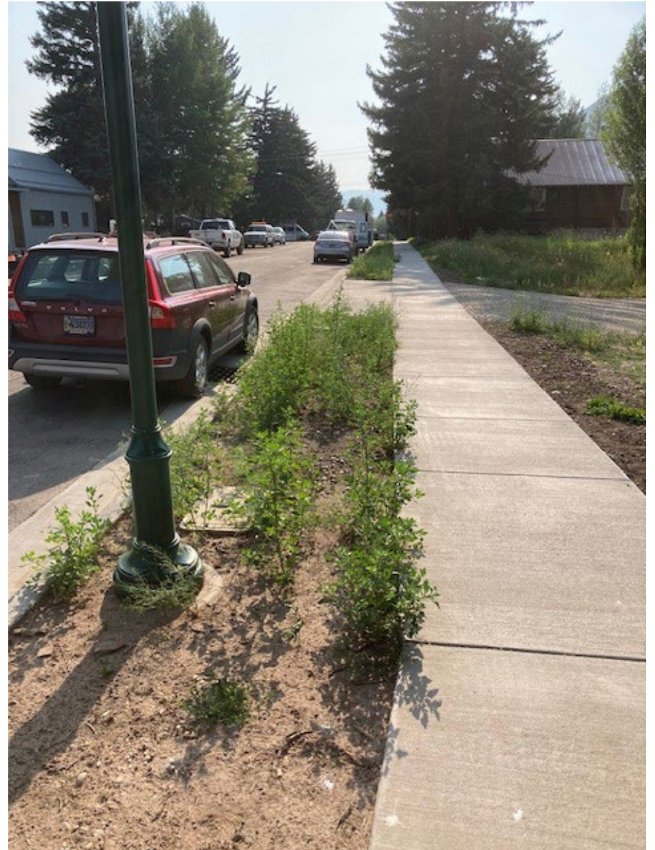
Kelly Ave sidewalk completed last summer
