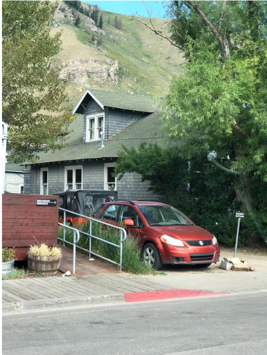
165 Glenwood South Elevation
