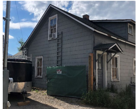
157 Glenwood North Elevation
