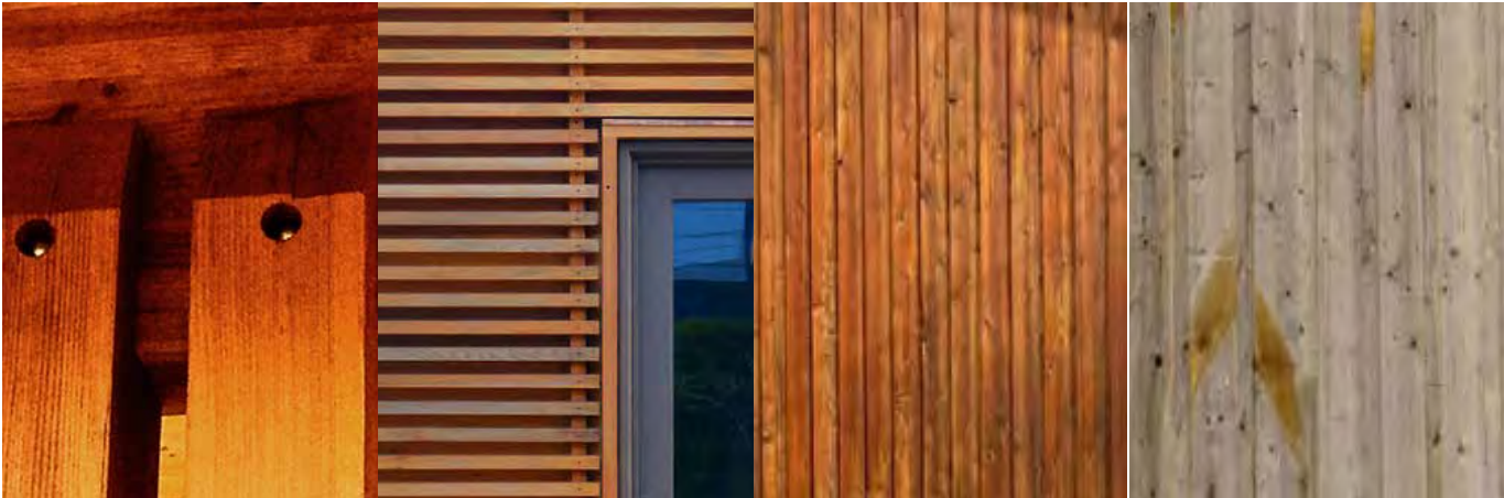
Timber Wood slat Vertical boards (stained) Vertical boards (weathered)
