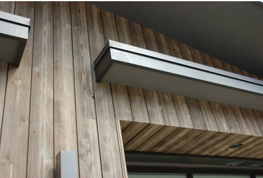
Example of wood siding wrapped to soffit surface
