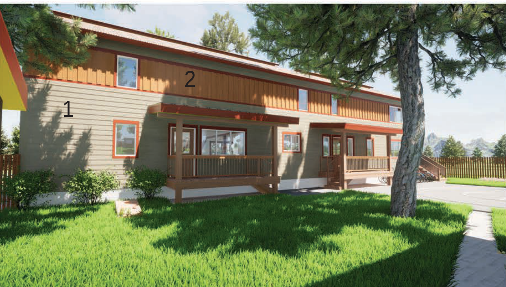
VAN VLECK - South Elevation view from courtyard
