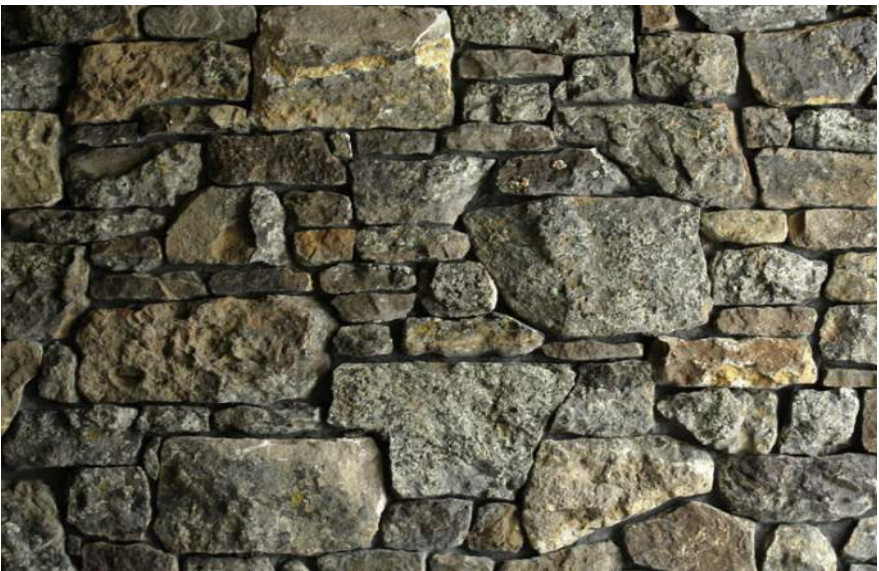
STONE (MONTANA MOSS ROCK - SELECT STONE) BUILDING WALL CLADDING AT LEVELS 1-2 PROJECTING BAYS
