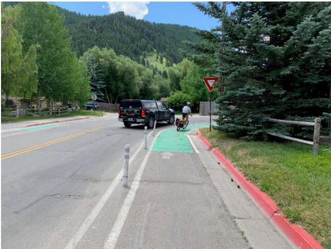
Figure 3 – Right turn pinch point squeezes cyclists
