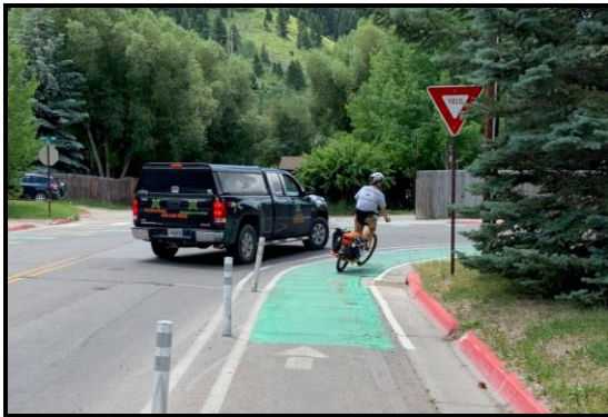
Pinch point on southbound Scott Lane turn onto Maple Way
