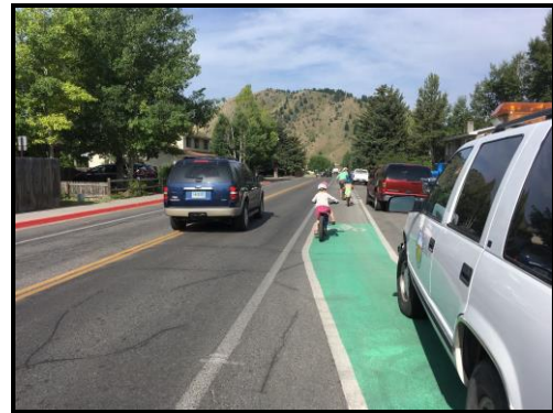
Un-protected, substandard-width, bike lanes on Maple Way
