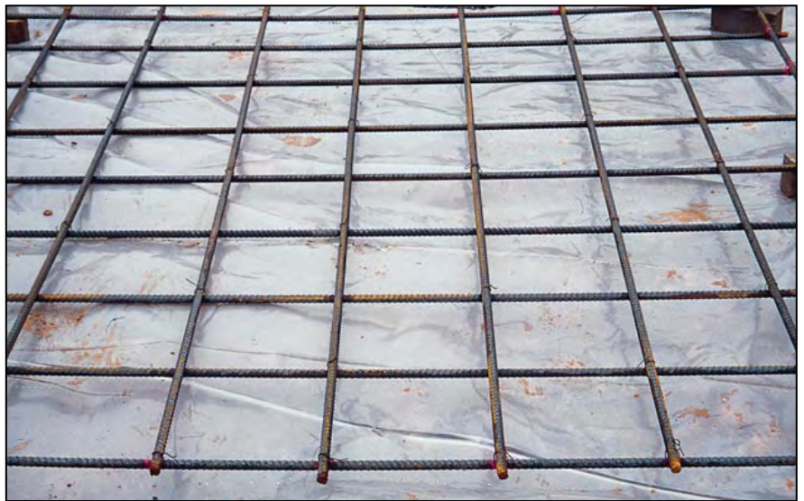
Rebar in concrete slabs placed directly on a vapor retarder help to control slab curling and cracking. Use supported deformed bars no smaller than #4, and space the bars far enough apart so workers can step between them.
