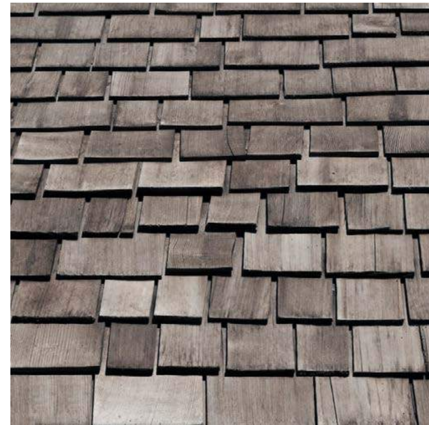
WEATHERED CEDAR ROOF SHINGLES
