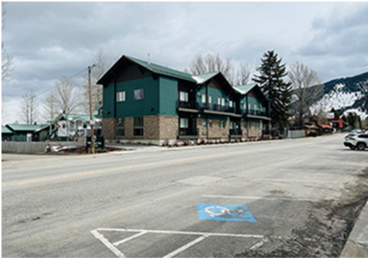
View towards E. Broadway Ave.
