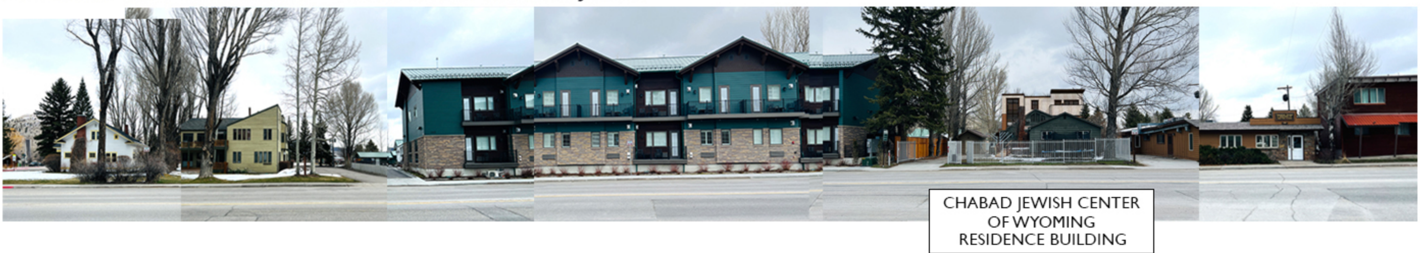
Street side view to the North - 211 to 325 E. Broadway Ave.
