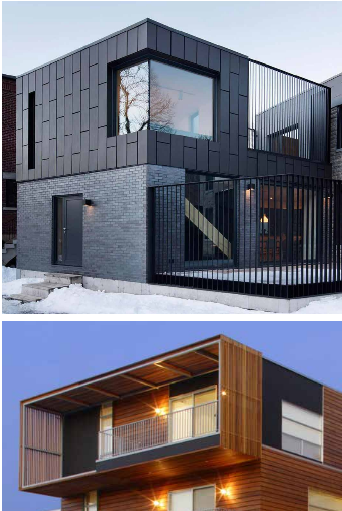
3 METAL PANEL RAINSCREEN EXTERIOR CLADDING @ WINDOWS & STAIRS
