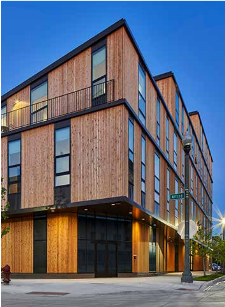
2 CEDAR SIDING EXTERIOR WALLS, LEVELS 2 & 3, & ROOF FASCIAS
