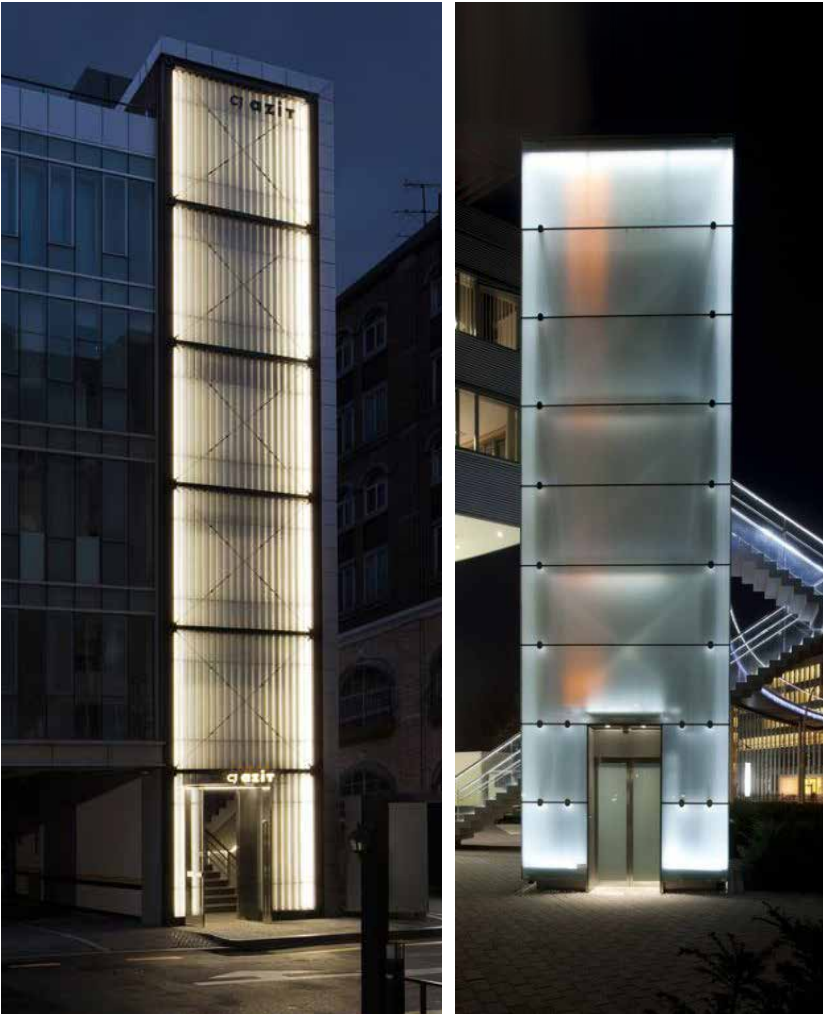
4 FROSTED GLASS / FRITTED GLASS STAIR TOWERS ALONG MILLWARD ST.
