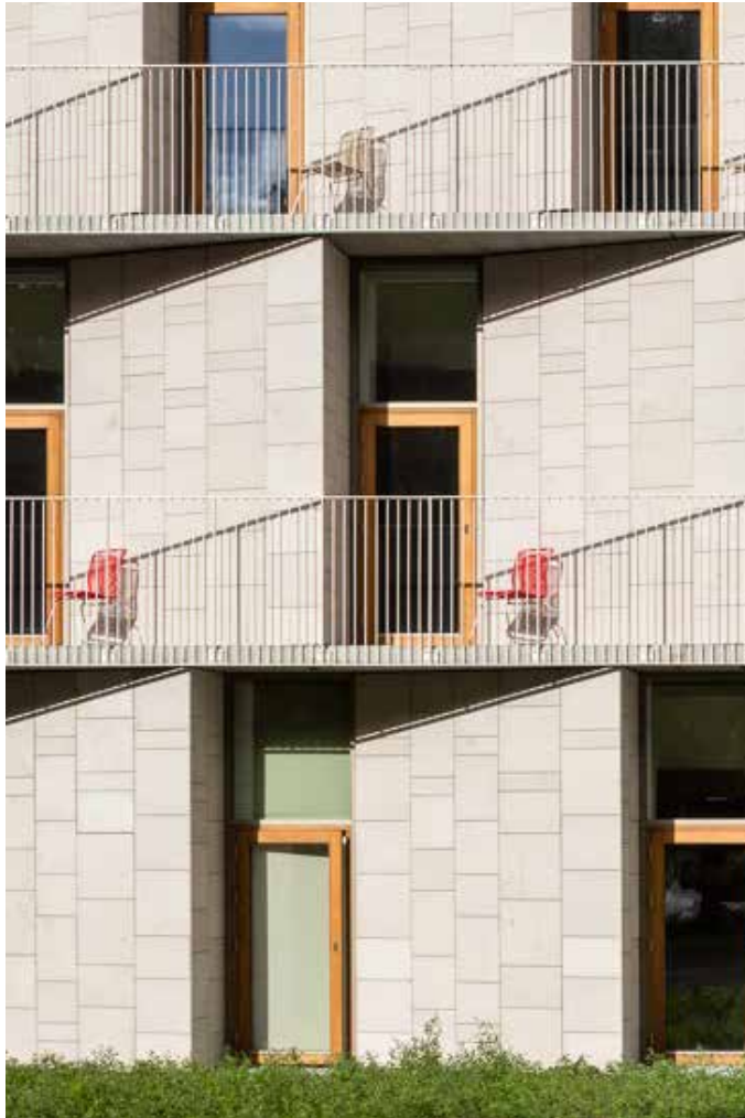
1 FIBER CEMENT PANELS EXTERIOR WALLS, LEVEL 1
