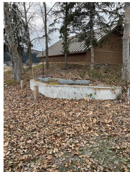
Photo 1.27. Cell 4 Water Control Structure
