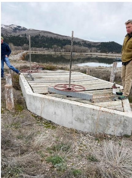
Photo 1.26. Cell 3A Water Control Structure
