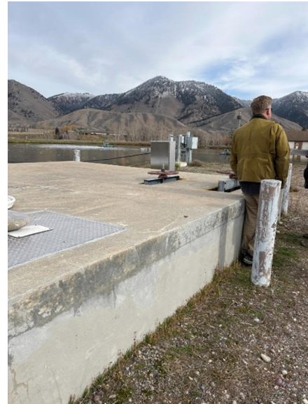
Photo 1.25. Cell 1 and 2 Water Control Structure
