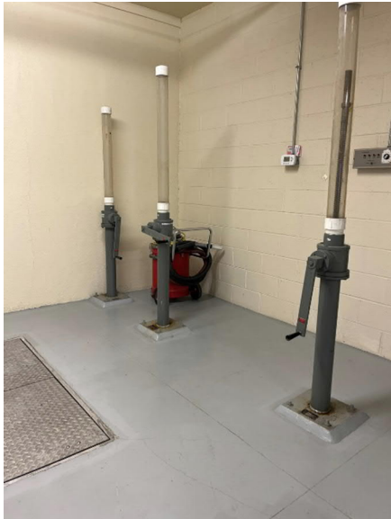
Photo 1.28. Cell 5 Water Control Structure
