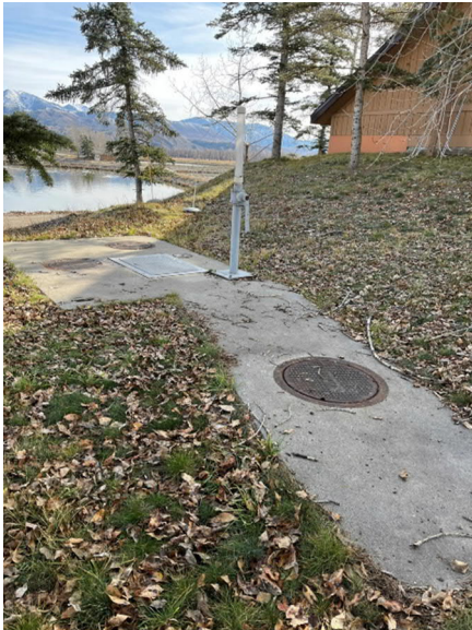
Photo 1.24. Influent Water Control Structure
