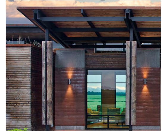
RUSTIC WOOD COLUMN WITH CARBONIZED STEEL COLUMNS
