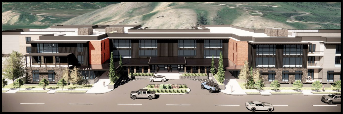
Mercill Avenue Pedestrian Entrance (south elevation):
