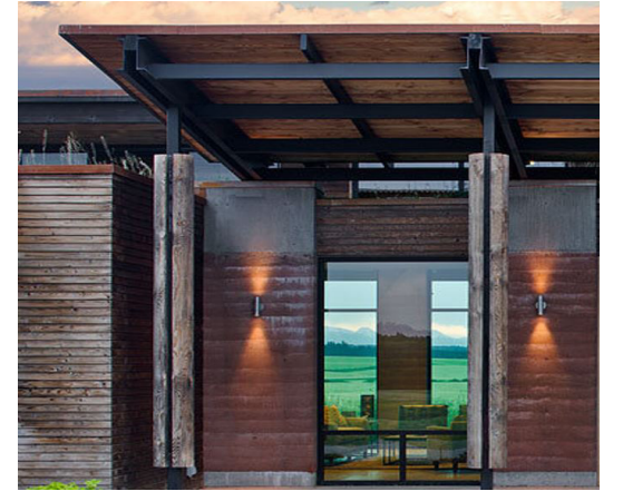
RUSTIC WOOD COLUMN WITH CARBONIZED STEEL COLUMNS
