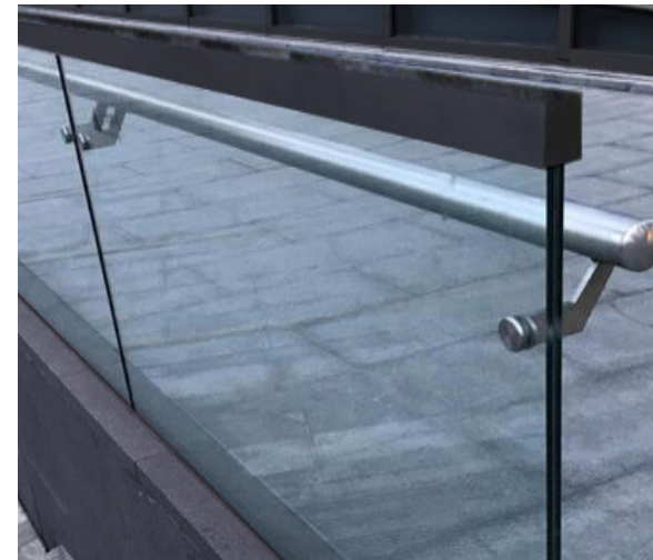
INDUSTRIAL STEEL / GLASS RAILING @ POOL AREAS
