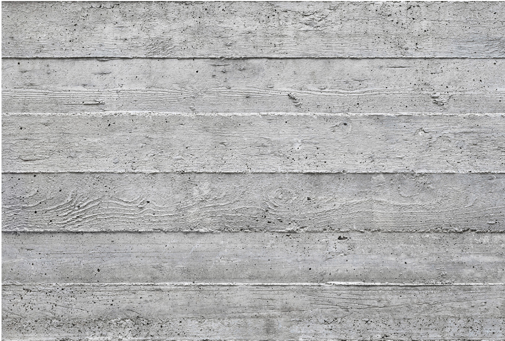
BOARD FORM CONCRETE BUILDING WALL CLADDING
