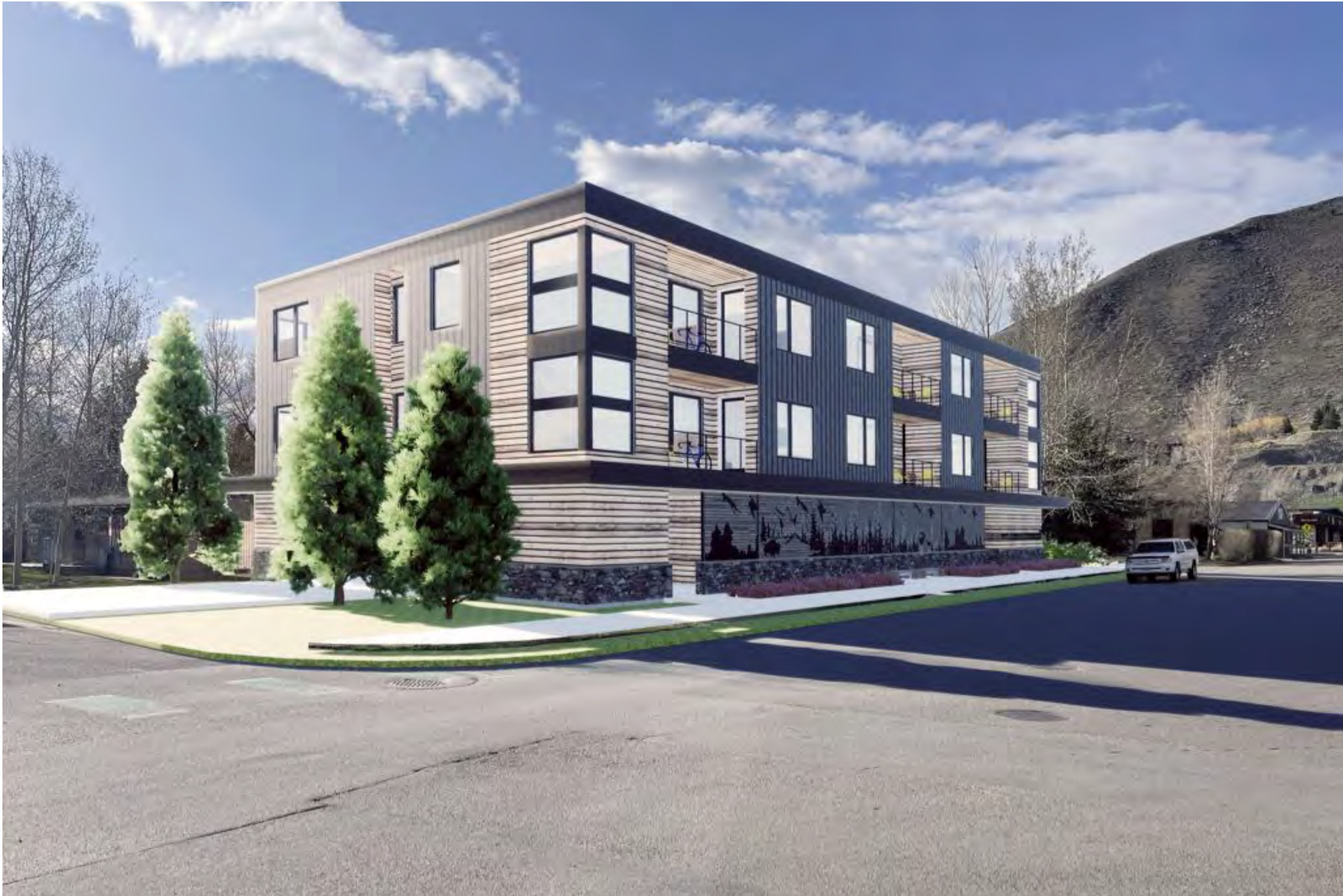
VIEW FROM THE CORNER OF SIMON LANE AND SCOTT LANE
