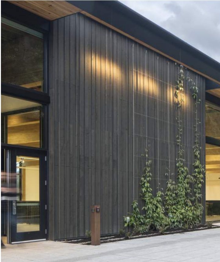
Charred Wood Cladding
