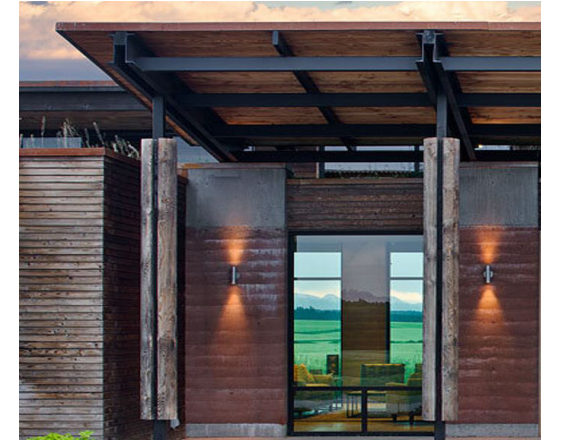
RUSTIC WOOD COLUMN WITH CARBONIZED STEEL COLUMNS
