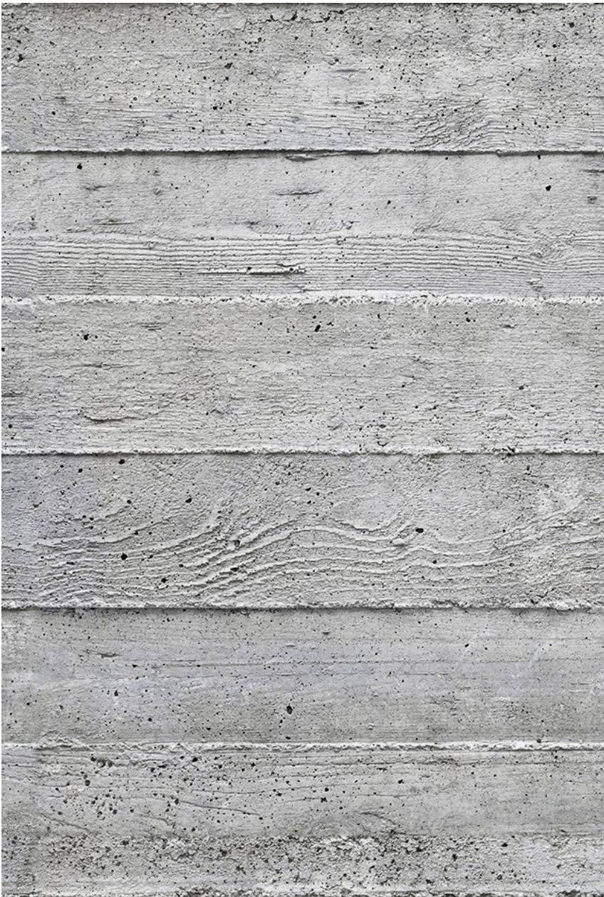
BOARD FORM CONCRETE FOUNDATION RETAINING WALLS
