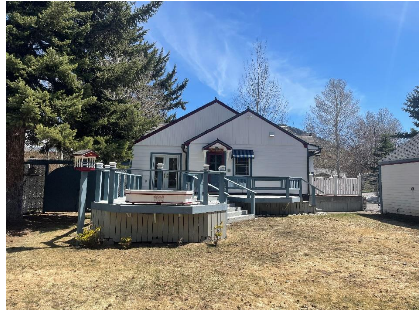
Rear elevation & deck
