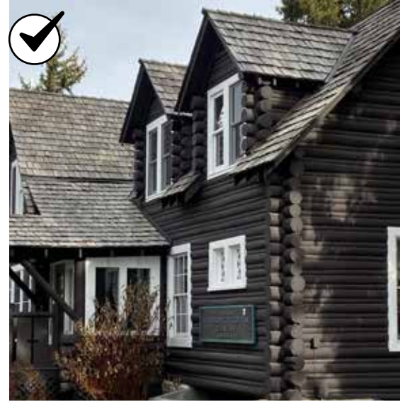
Preserve original building materials.
