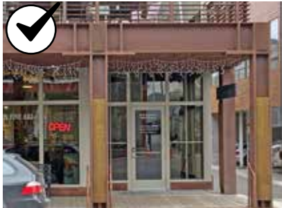
Area 1 & 2 Covered walkway
