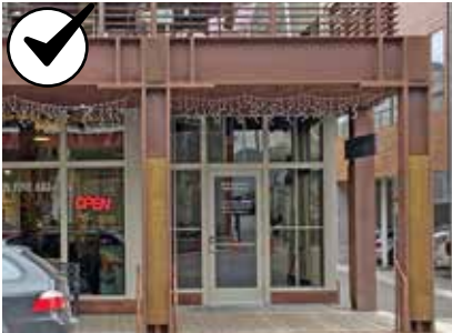
Area 1 & 2 Covered walkway
