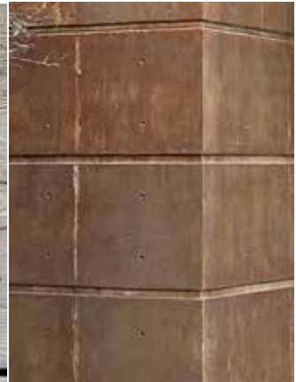
Formed concrete (colored blocks)
