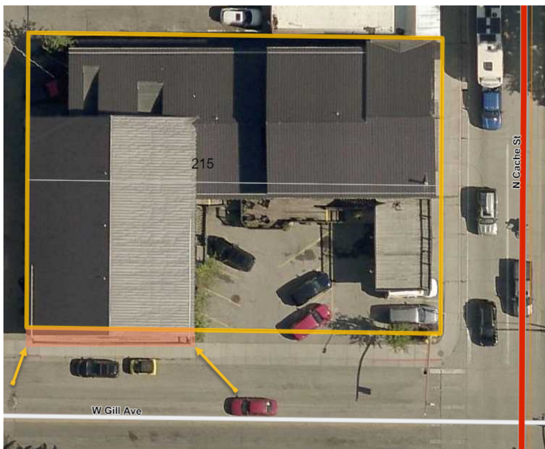
Figure 1. Aerial image of the property showing the existing encroachment highlighted between the two arrows.
