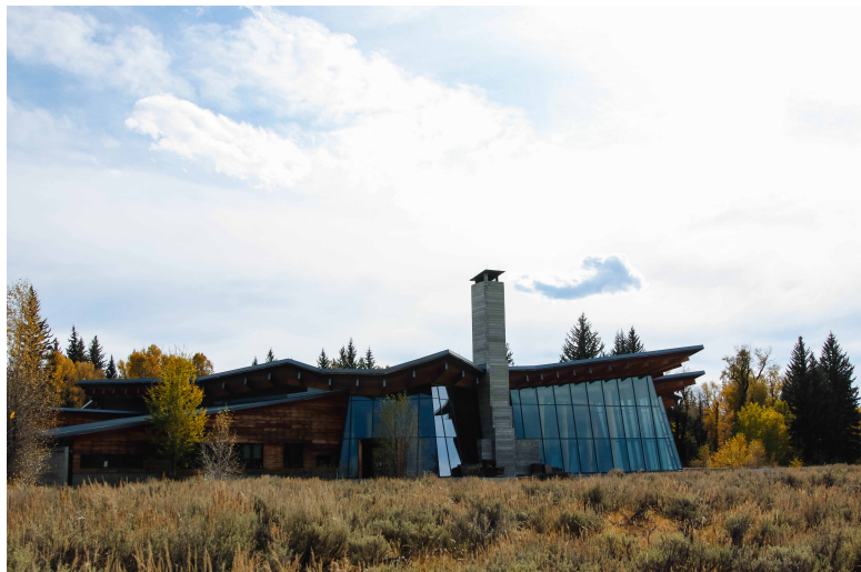
VISITOR CENTER-BUILDING A, D
