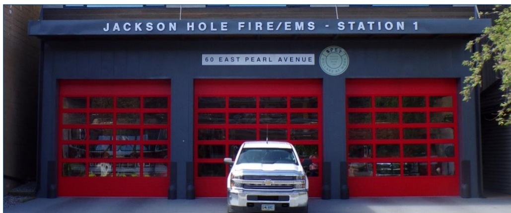
Figure 26: Jackson Hole Fire/EMS Station 1
