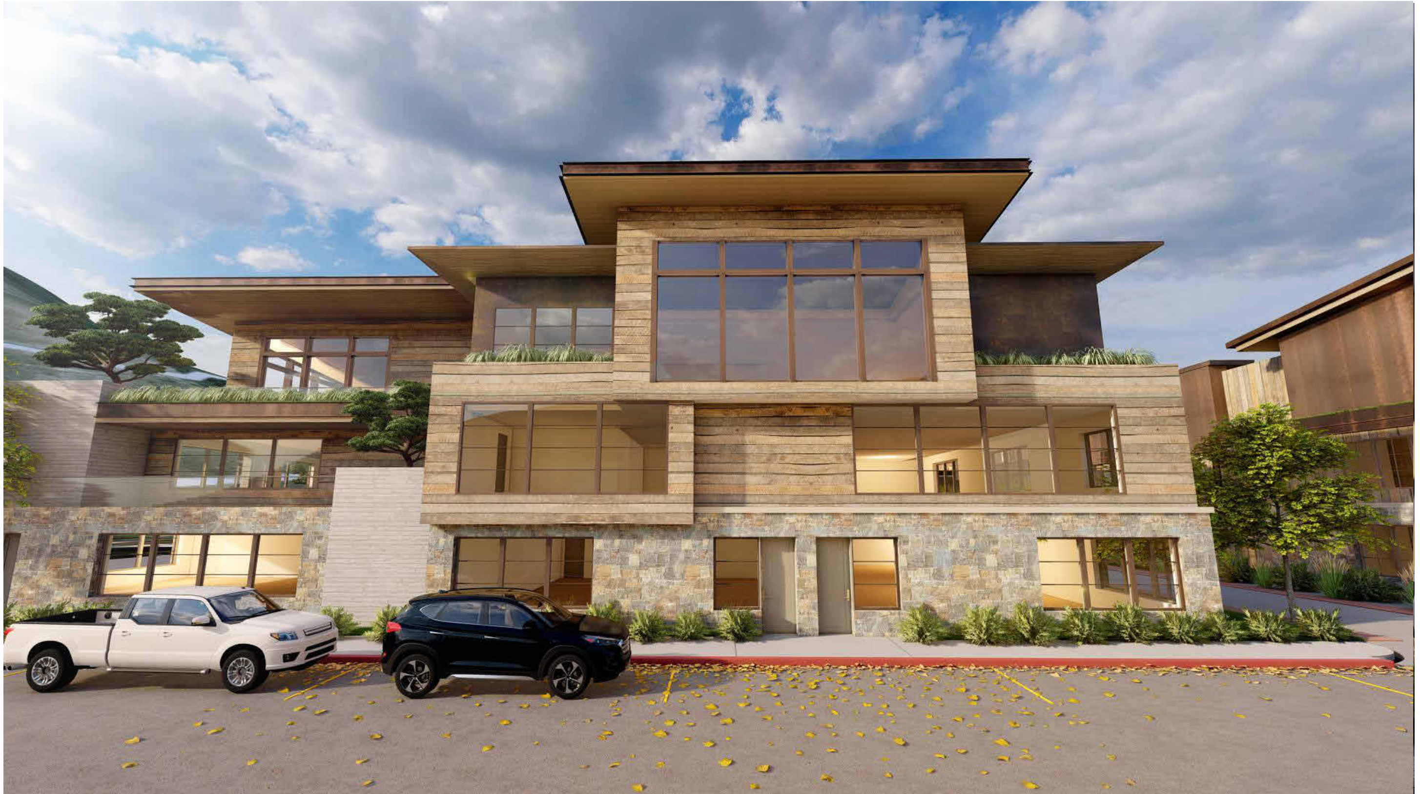
BUILDING A FROM SOUTH
