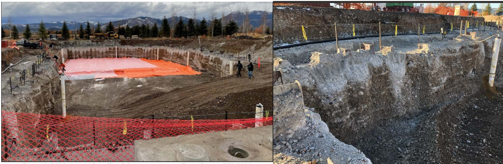
Figure 1: DSM secant pile wall and dewatering system. Teton County, WY (2020)
