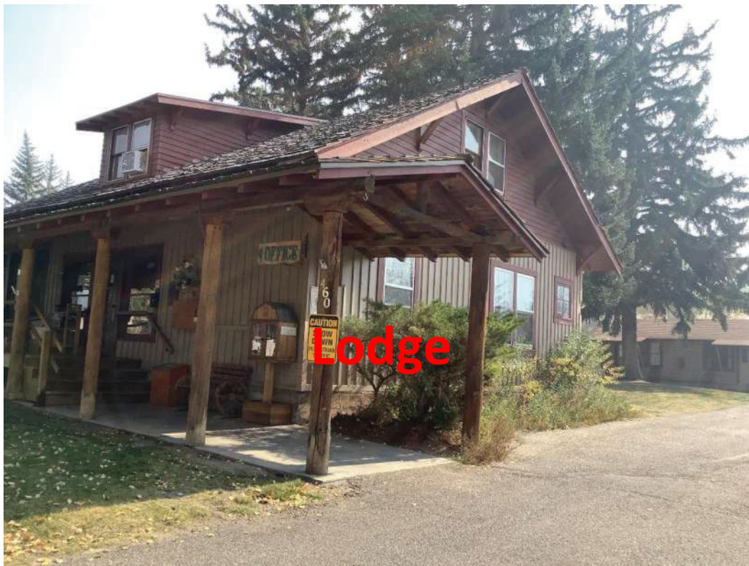
Photo 10 - Photo Point 9. Office building for Hitching Post Lodge with upstairs employee housing unit and basement storage (October 15, 2024).
