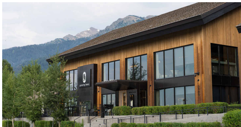
GRAVITY HAUS-BUILDING D
