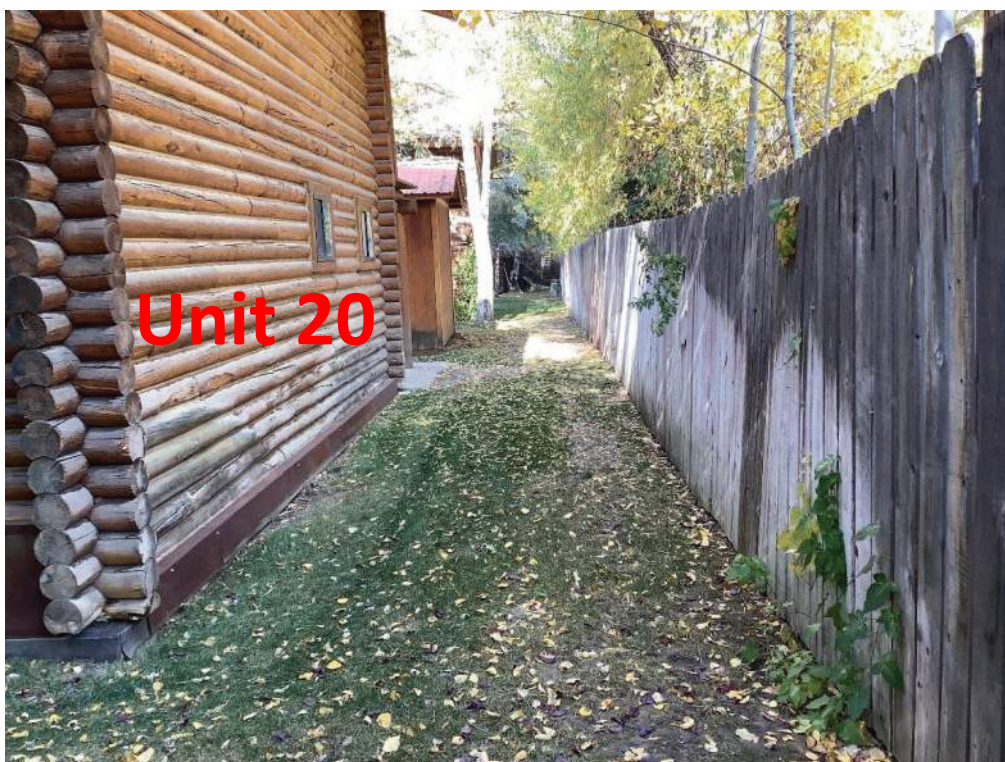
Photo 6 – Photo Point 3. View from southeastern corner of Subject Property looking north (October 15, 2024).
