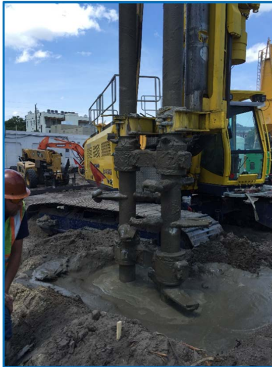
Deep Soil Mixing
