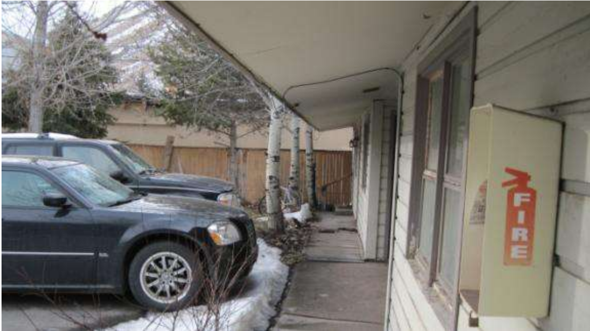
A view of the front covered porch
