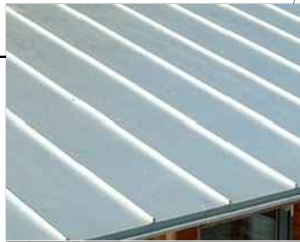
WEATHERED ZINC STANDING SEAM METAL ROOFING
