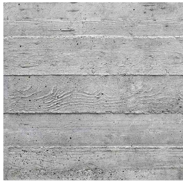
BOARD FORM CONCRETE PROJECTED BASE
