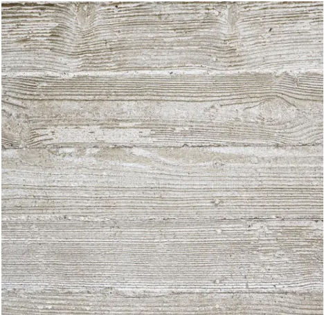
BOARD FORMED CONCRETE
