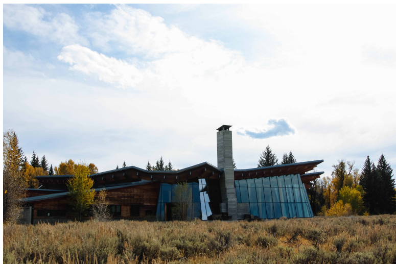
VISITOR CENTER-BUILDING A, D
