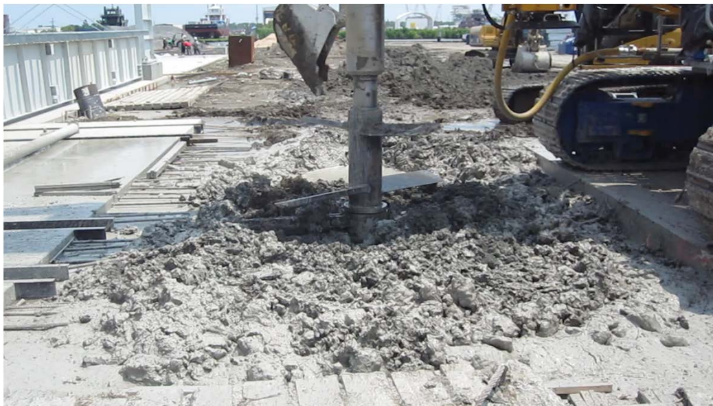
Deep Soil Mixing
