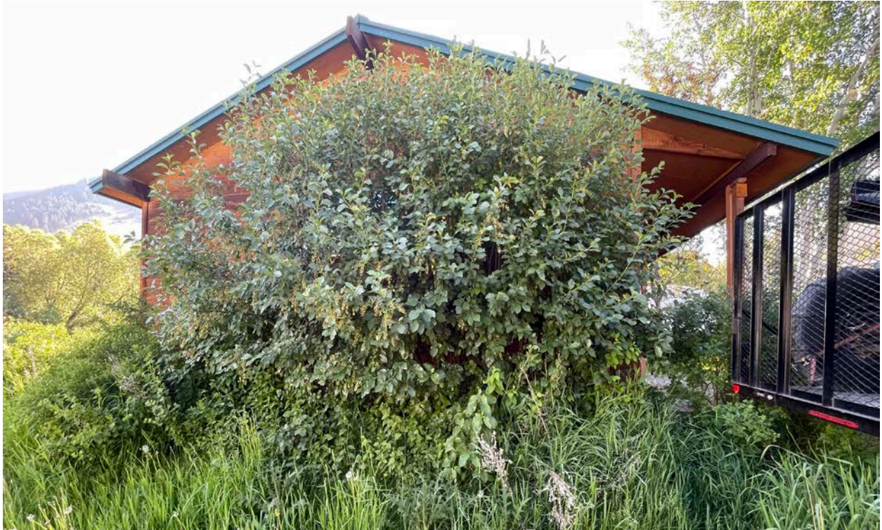
Existing structure, West façade
