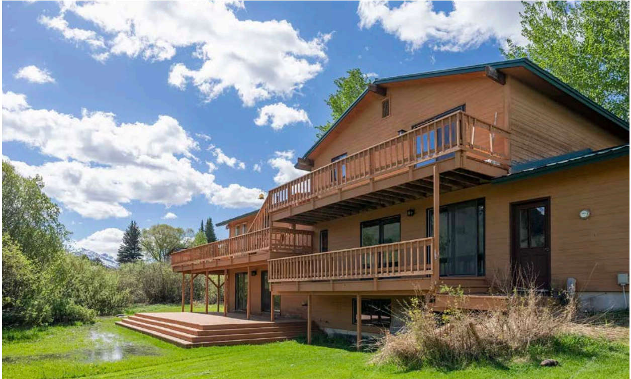
Existing structure rear façade
