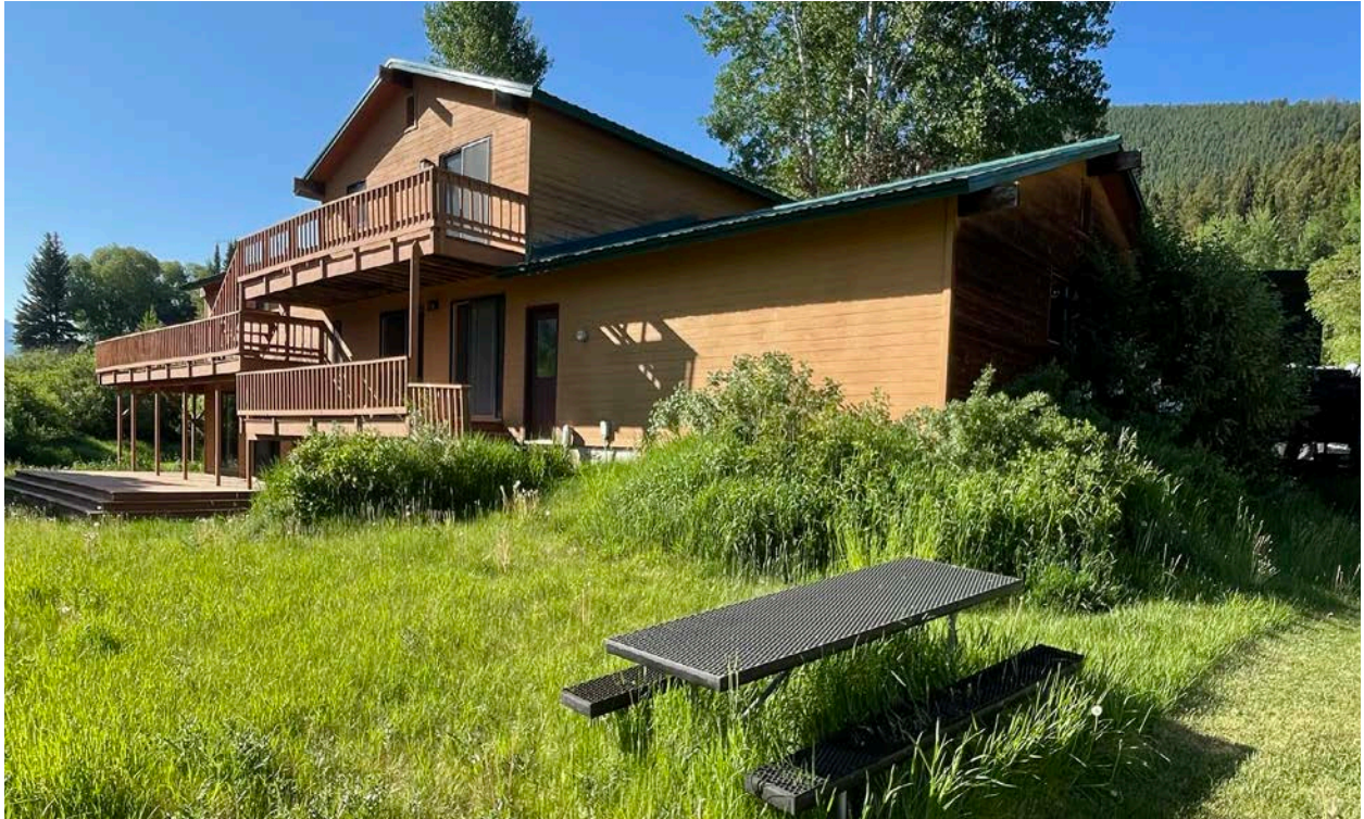
Existing structure NW corner
