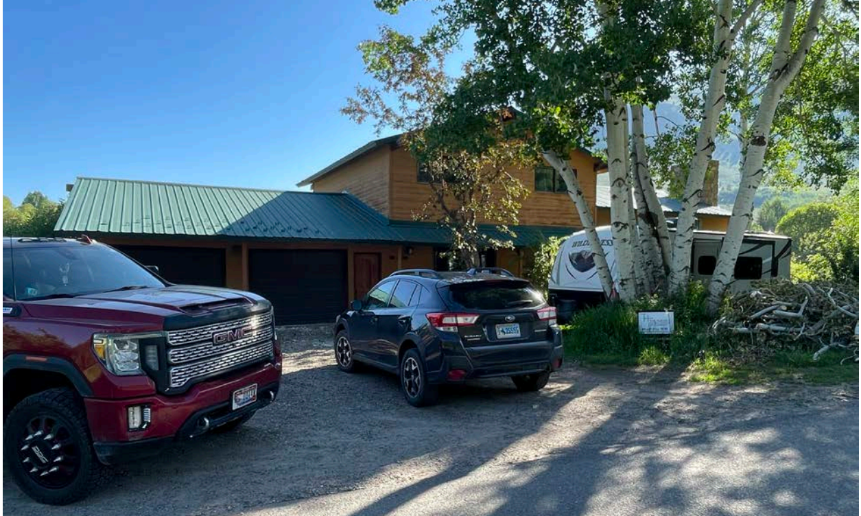
Existing structure street view
