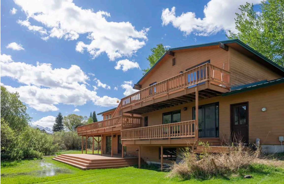
Existing North Facade
